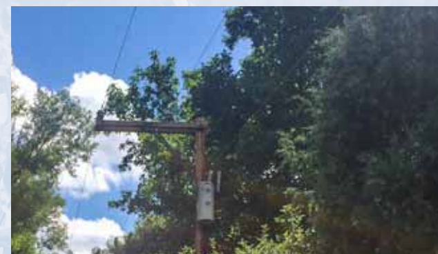
Currently, we trim away vegetation to a distance of at least 10’ from lines & equipment. This way, we only need to revisit an area once every 3 years.
