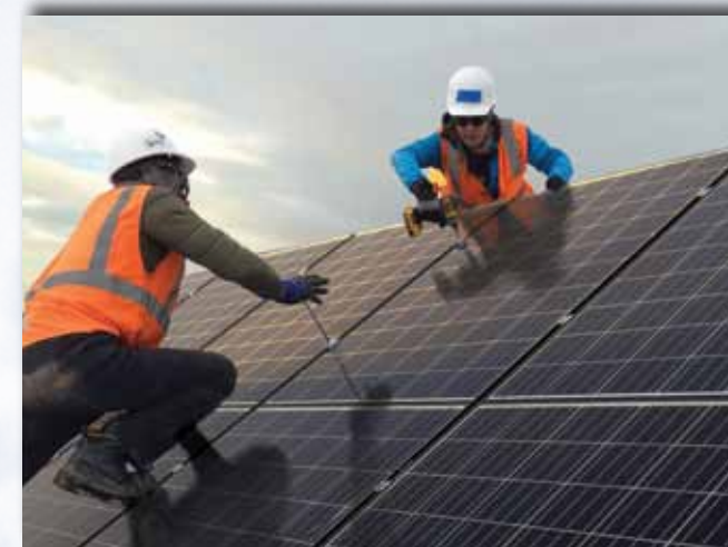
Completed by volunteers in 2016, the I.Q. Solar Array, in Norwood, CO is providing solar energy to members who could not afford to build their own array, but who can use the affordable power to help ease the burden on their budgets.
