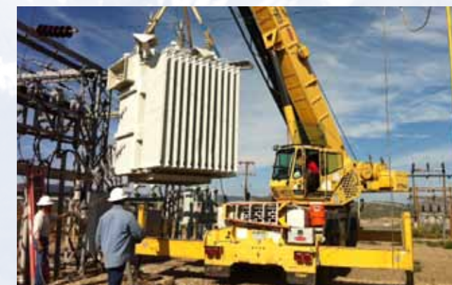
The new Nucla Substation Transformer will serve the needs of the Nucla / Naturita area for many years to come.
