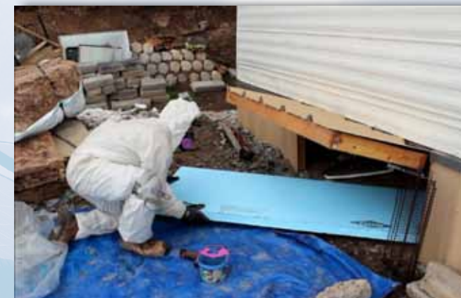
Home efficiency upgrades like this crawlspace insulation project can be completed at no cost to the member. Members save money every month, because their homes require less energy to keep them comfortable.
